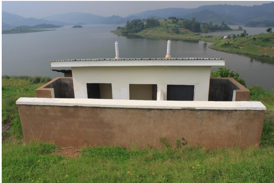
Figure 2: PVC Solar Chimneys on an outhouse at a school on Lake Bunyonyi
