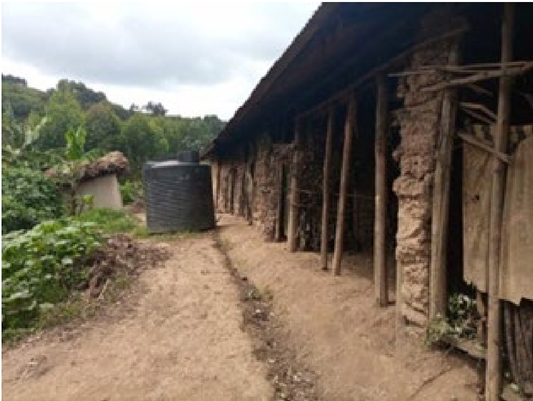
Figure 22: Ishunga Settlement Broken Water Tank
