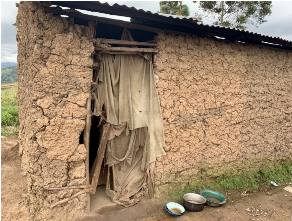
Figure 14: Batwa Semi-Permanent House with Iron Roof
